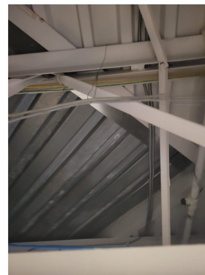
CORNER OF EXISTING SKYLIGHT OPENING - WHITE PAINTED DECKING & TRUSS TO STAY, DEMO SILVER DECKING CAP
